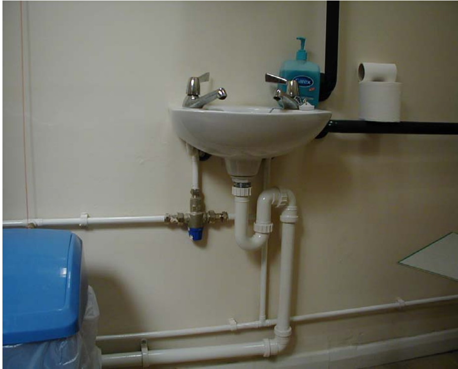
Disabled toilet on ground floor Note the Type 3 TMV which does not function properly
